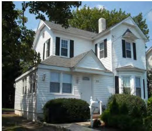
Oxford House – Cardinal Court Long Branch, New Jersey
